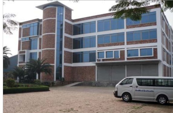
An OBL Financed Corporate Office Building
