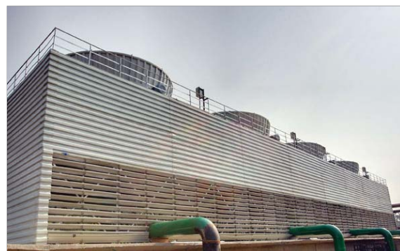
An OBL Financed Power Plant Project
